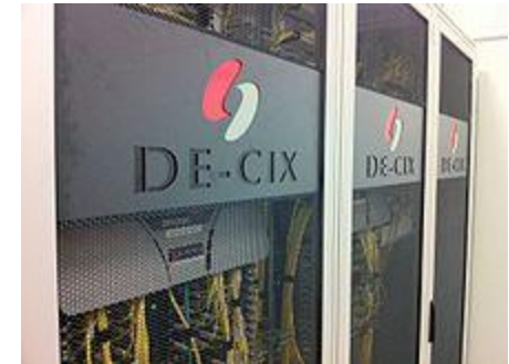
A 19-inch rack used for switches at the DE-CIX in Frankfurt, Germany
