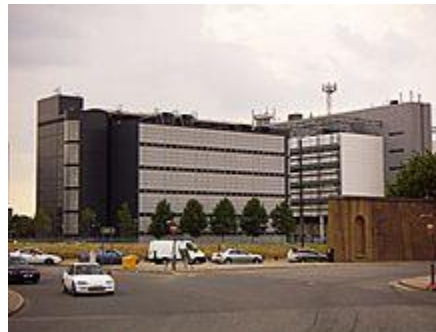
Main building of the London Internet Exchange (LINX)
